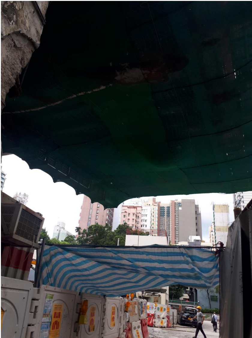
Figure A1: Impervious sheeting was added at the base of bridge at P6 site area.
